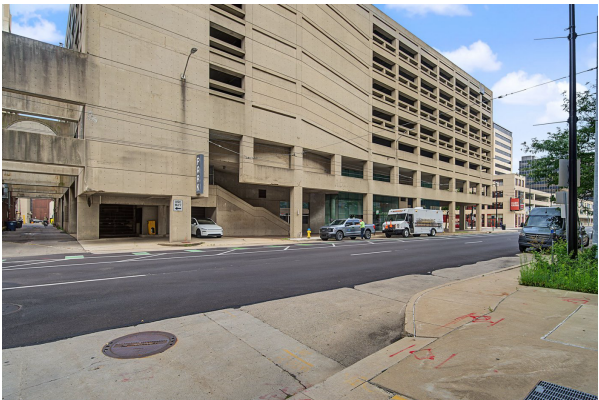
Attached parking garage
